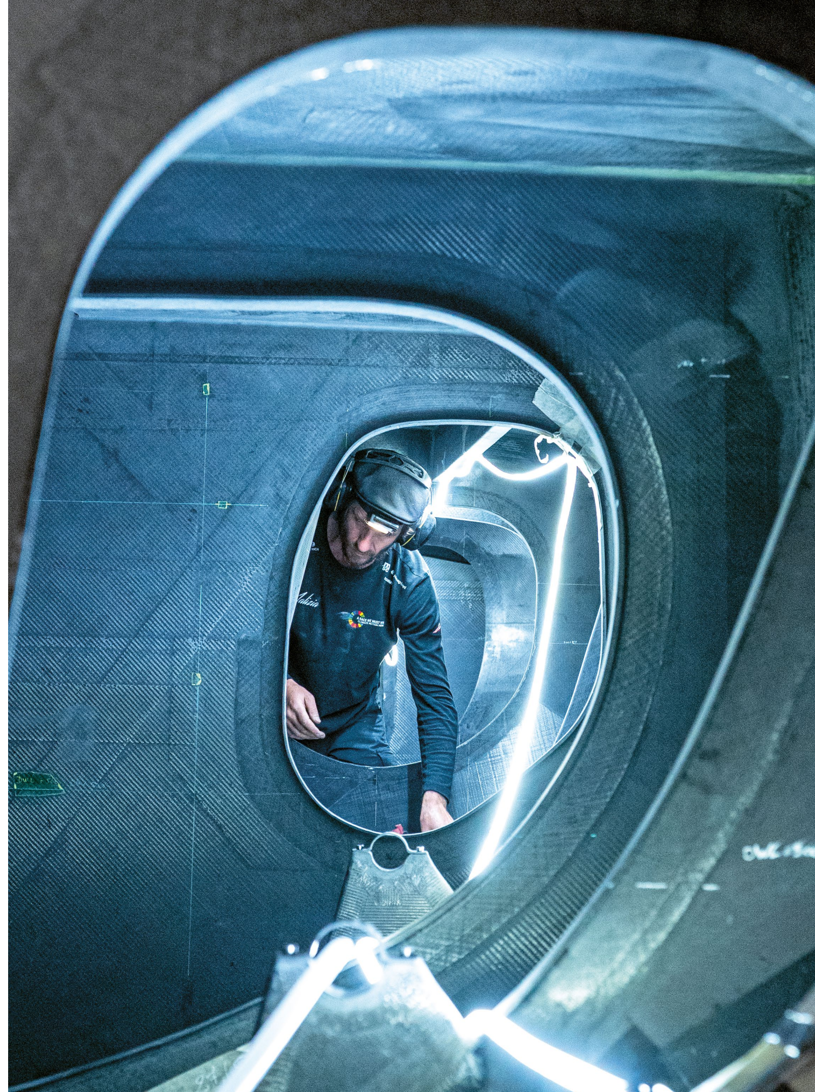
Early in the build, a technician examines Malizia 4's structure from the inside
